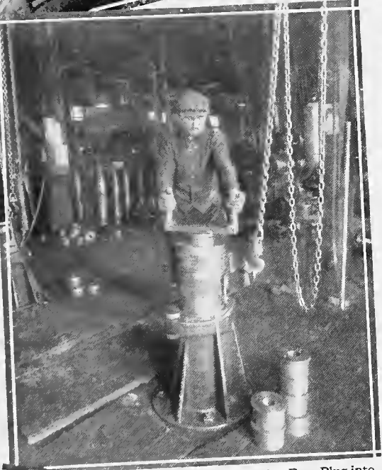
Screwing Base Plug into 10-Inch Shells
